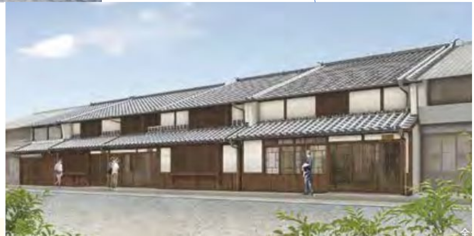
Accommodation utilizing the townhouses attached to the former Kanda family (in Okayama Prefecture) 2
